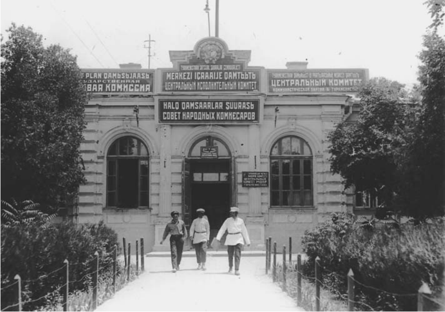
Figure 8. Building housing the offices of the Turkmen republic’s Council of People’s Commissars, Central Executive Committee, and KPT Central Committee, Ashgabat, 1930. Note misspelling of the Russian word “commissars.” (From the collection of the Russian State Archive of Film and Photographic Documents at Krasnogorsk.)
