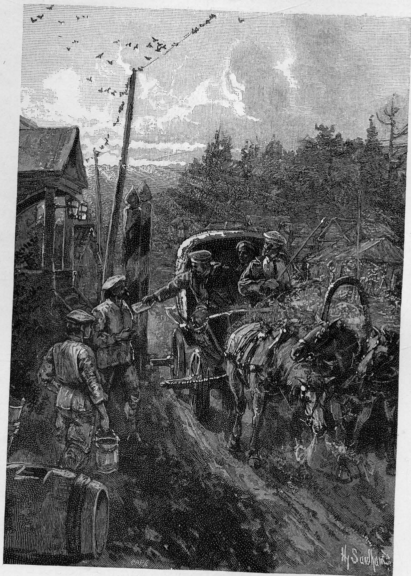
TÁRANTÁS AT A POST STATION.
